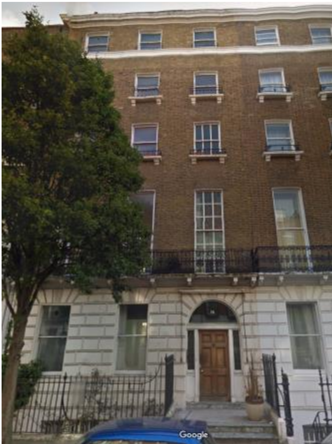
Front elevation of application site
